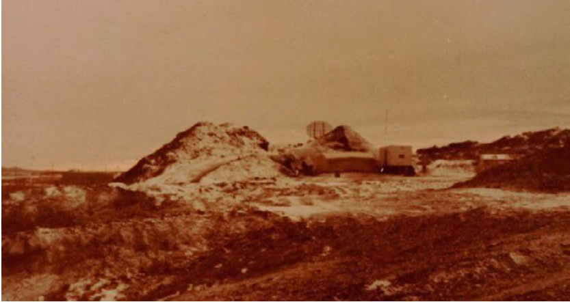
Radar TPS-43 Westinghouse, Río Grande (1982)
