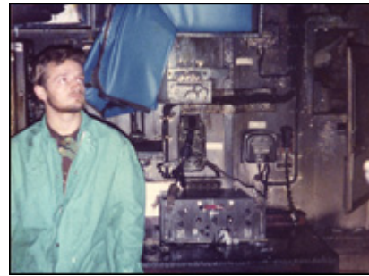
Tony Groom, at work in the boiler room
